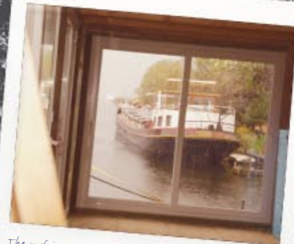
The roof is on and all windows and doors are in place. Now we need have no worries about the bad weather.
